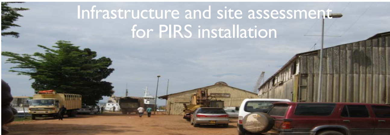
Port Bell, Kampala site inspection during an assessment for the installation of PIRS
